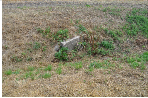
Plate 34 Field drain outfall
