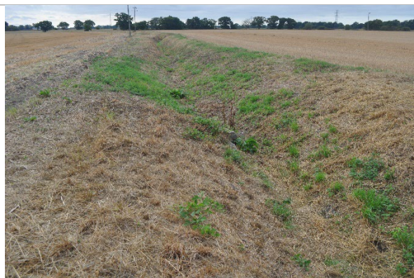
Plate 31 Trapezoidal nature of the channel at the upstream end of the reach
